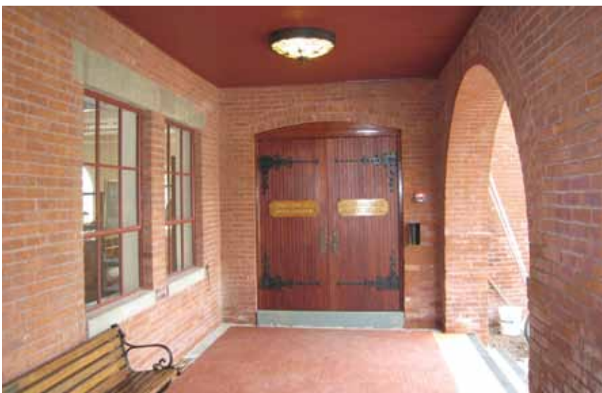
The entry at Ely Hall after restoration now features refurbished windows.
