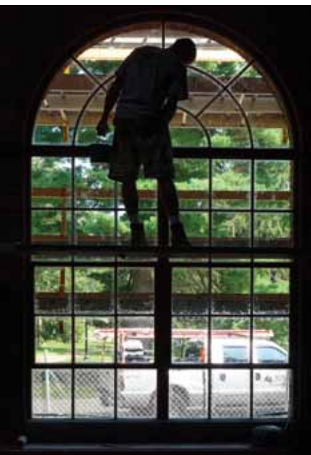
A Seekircher worker paints one of the windows at Ely Hall.
