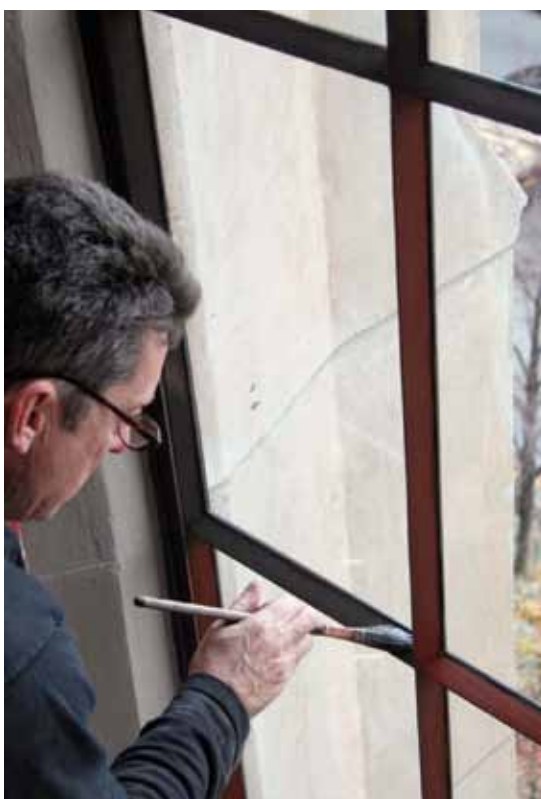
The final step at the Columbia University Hospital project in New York City was painting the windows. Ralph Whitehead of Seekircher applies two coats of paint.
